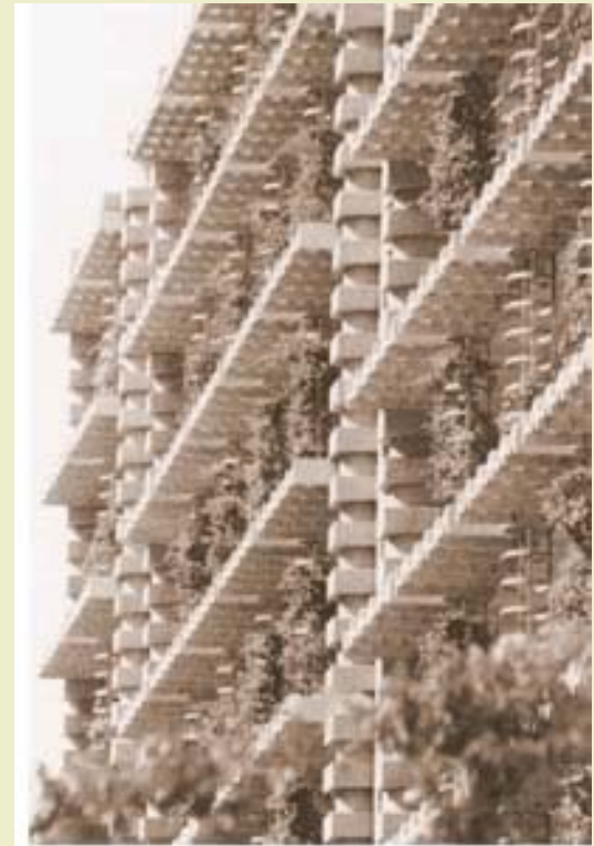
Eastgate building in Zimbabwe designed by Mick Pearce, based on termite hills
